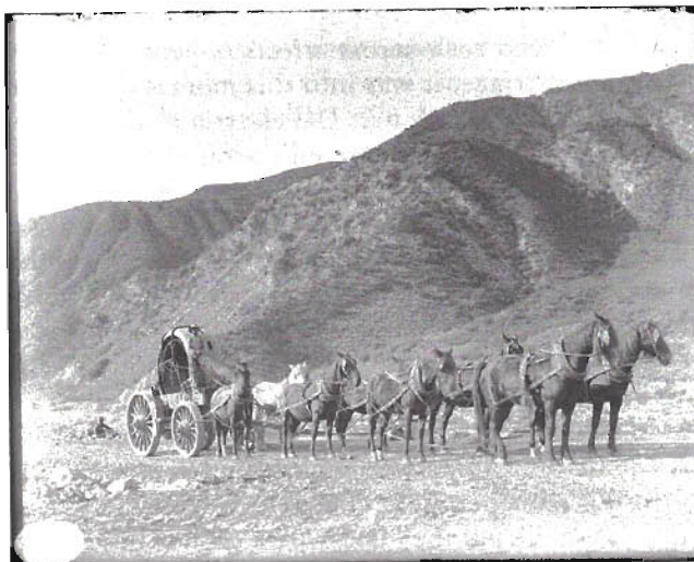
Figure 3.1 A horse team hauling the first generator to the Mill Creek #3 Hydroelectric plant, California ca. 1903. Reprinted courtesy of The Huntington Library and the papers of Southern California Edison.
